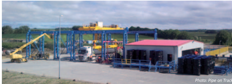
Photo: Pipe on Track
