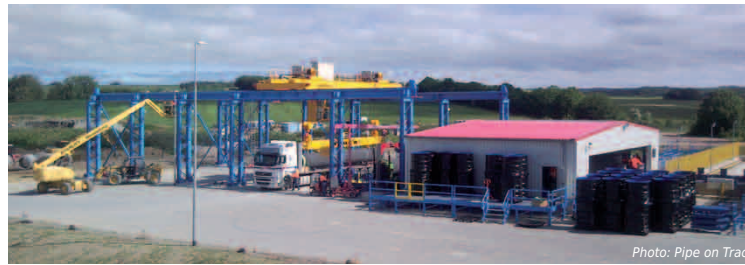
Photo: Pipe on Track
