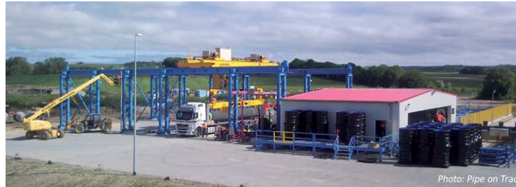
Photo: Pipe on Track
