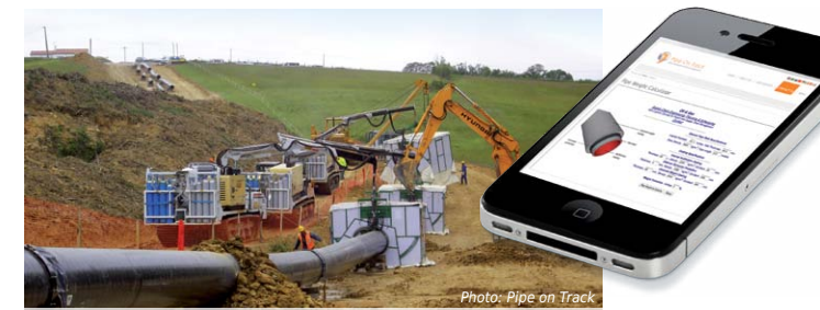
Photo: Pipe on Track
